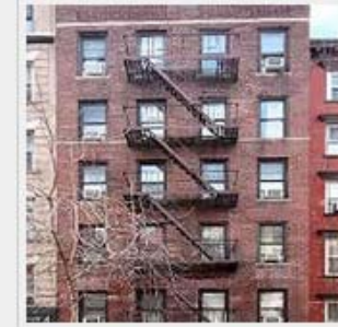
278 East 10th Street & 78 East 3rd Street NY
